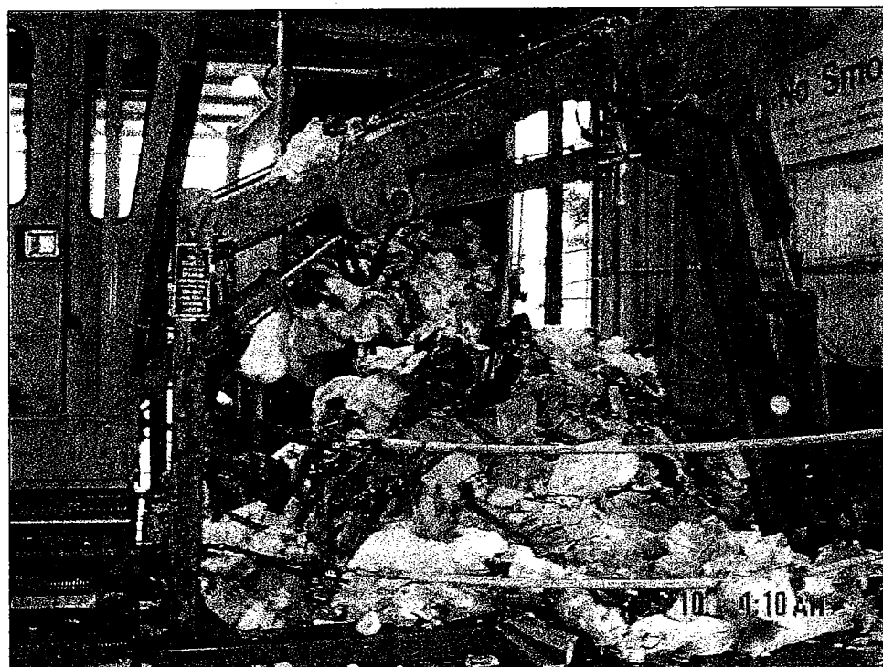
Garbage can overflow and fall onto the area across the dumping chute.
